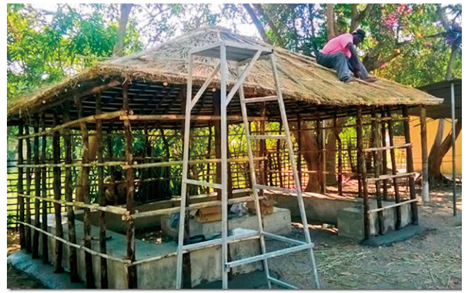
Renovation of arbor
