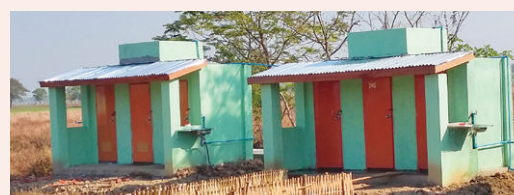
Completed school toilets
