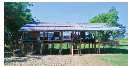
Temporary school building villagers built
