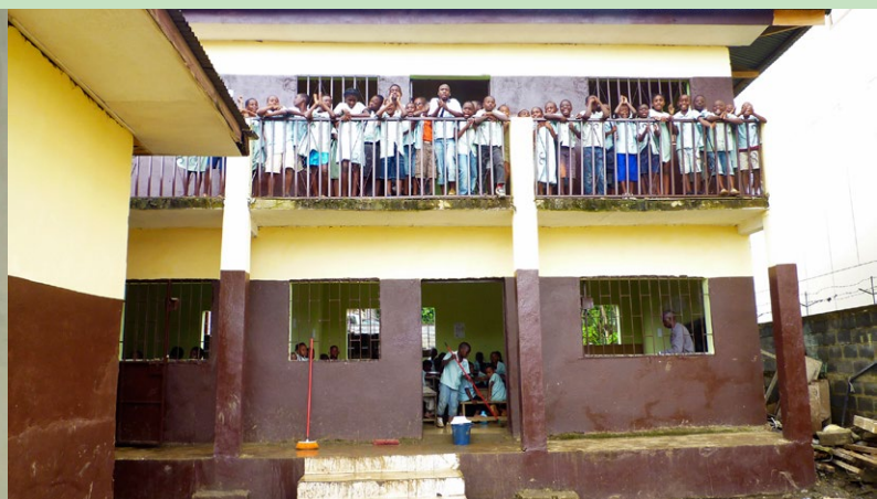
New school building
